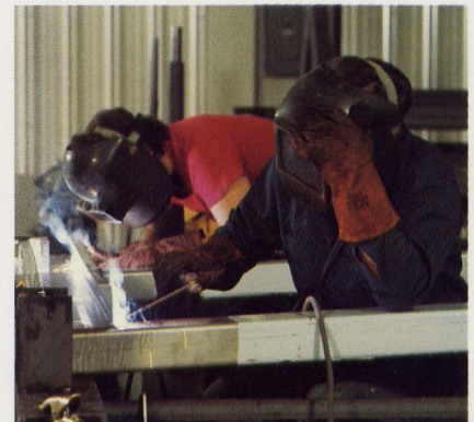
Welding vertical support structures.
