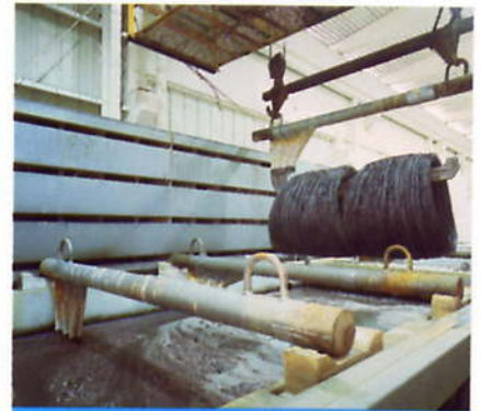
H 2 SO 4 pickling tanks in operation.
