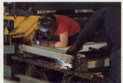
Fabricating vertical members in welding jig.
